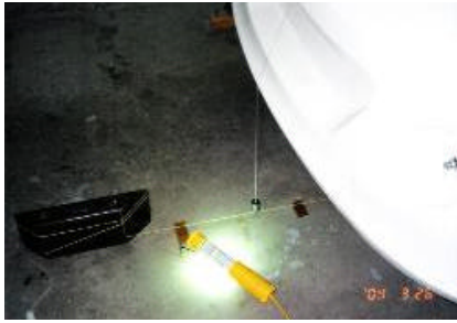
Hood & frame center lines aligned during body panel adhesive bonding process.
