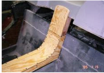
Final console substrate fabricated in plywood.
