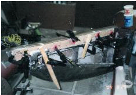
Forming upper door trim panel substrate to curved door flange using "partial kerfs" and epoxy putty to "freeze" the shape.
