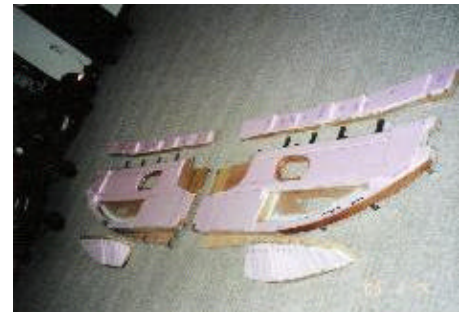
Door trim panel substrates with polystyrene foam adhesively bonded in place prior to shaping and smoothing.
