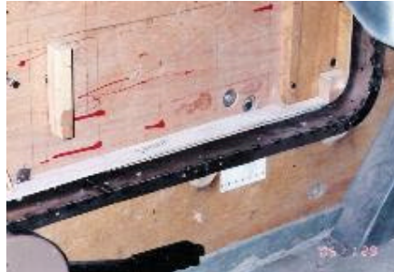
Door sill upholstery substrate with flange skip welded in place.
